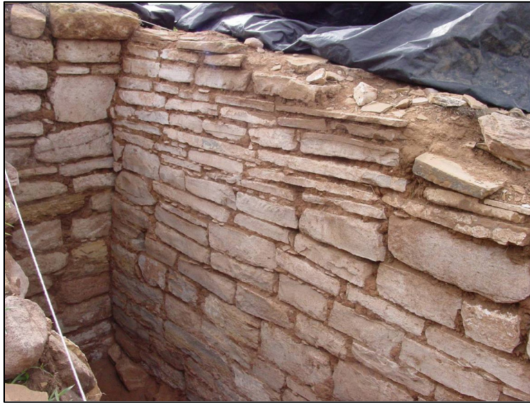
Figure 5.6. Core-and-veneer-like masonry with chinking stones, Structure 140 east exterior wall, Albert Porter Pueblo.
